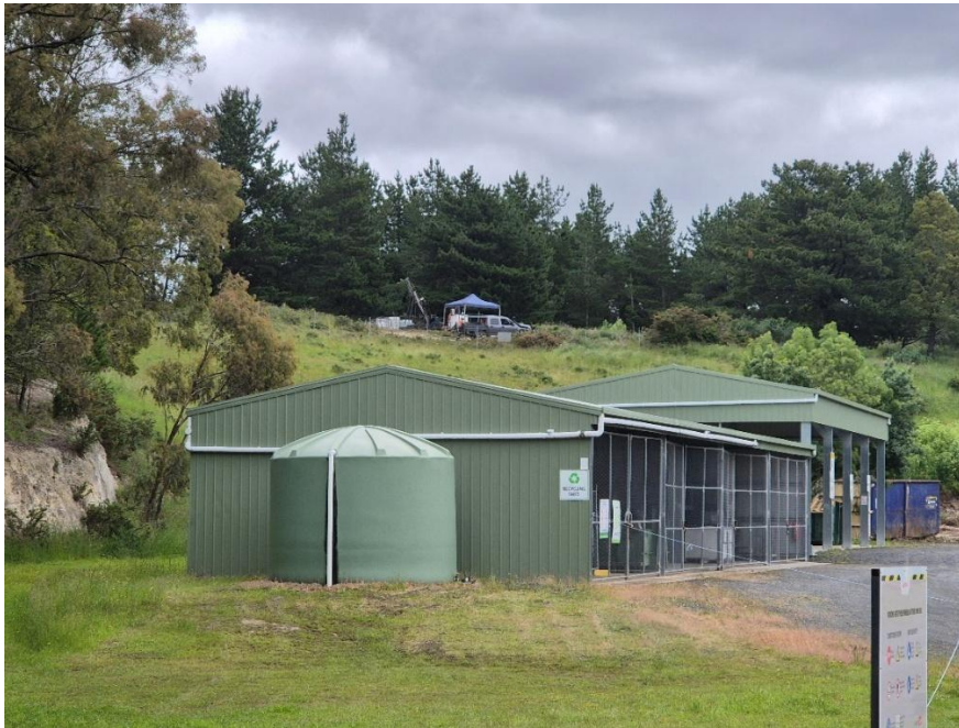
Figure 4: Drill rig on hill behind Mt Egerton Waste Transfer Facility - which sits in the filled-in historical open cut gold mine ("Quarry Lode") 1 .
