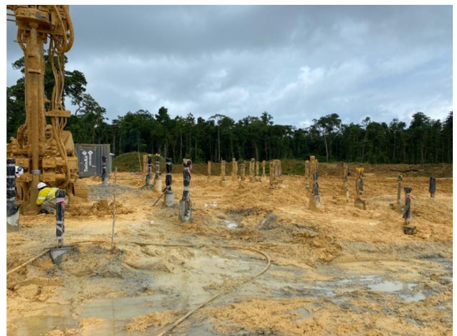
SAG / Ball Mill Micropiling Foundations
