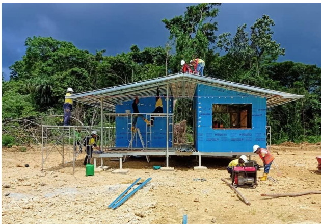
Figure 3 Shows the construction of the new elevated steel framed houses. Modern methods are being used to replicate as much as possible the traditional style of the village houses.
