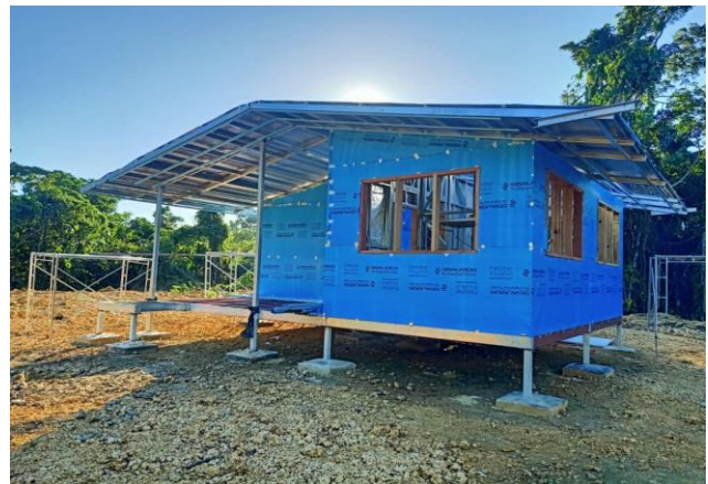
Figure 3 Shows the construction of the new elevated steel framed houses. Modern methods are being used to replicate as much as possible the traditional style of the village houses.
