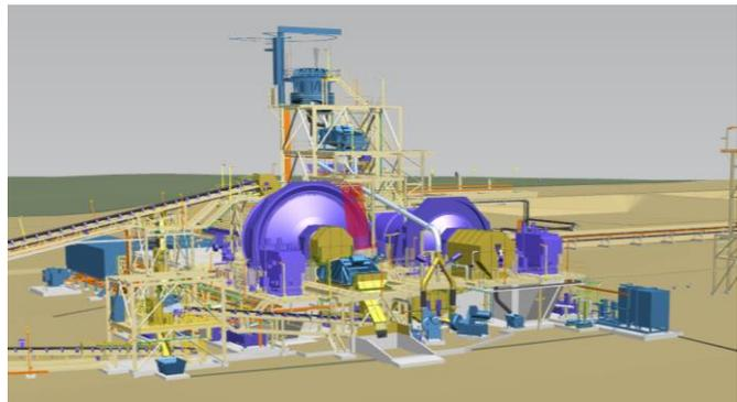
Figure 4: GR Engineering-designed 2.4Mtpa gold process plant
