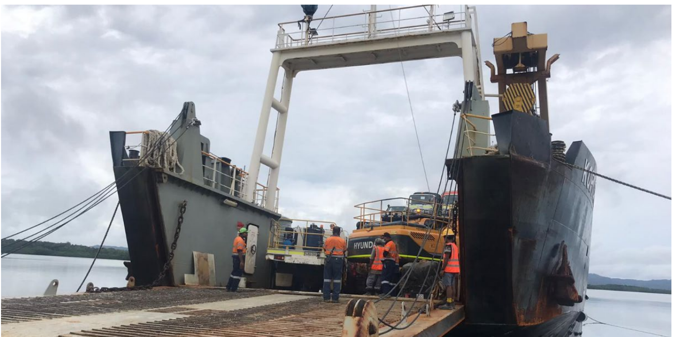
Figure 1: Equipment mobilised to site to continue the Civil Works Program
