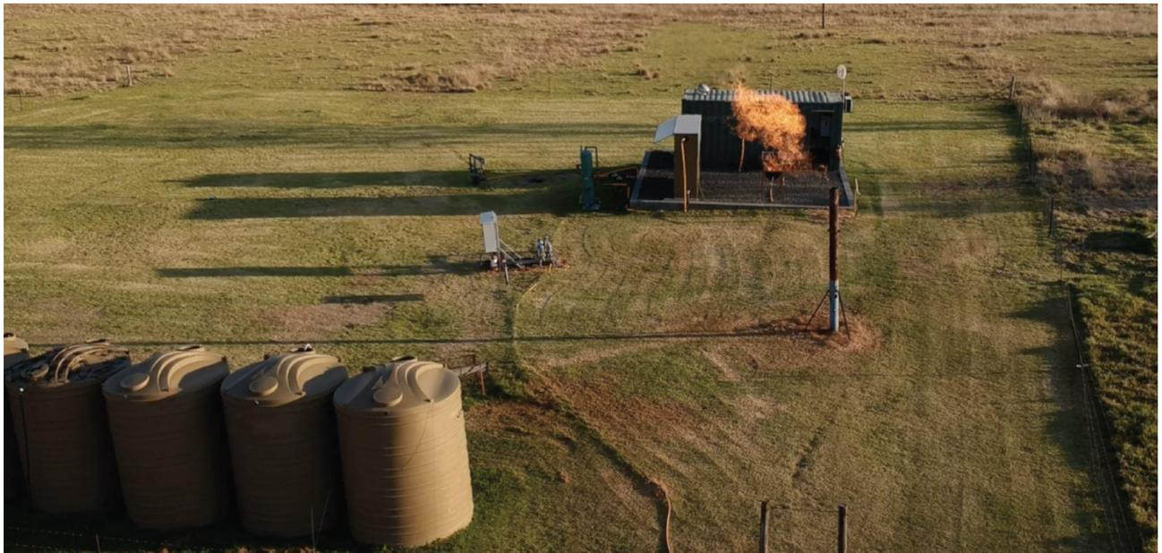
**Figure 3 - Pilot production well KA-03PT flaring gas at Amersfoort Project**
