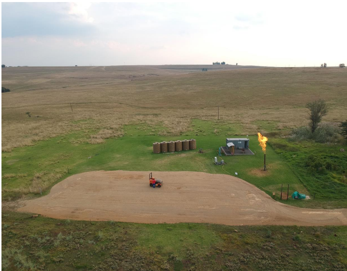
Figure 1 –Completed upgrade to road and terminal landing with flaring Well KA-03PTR
