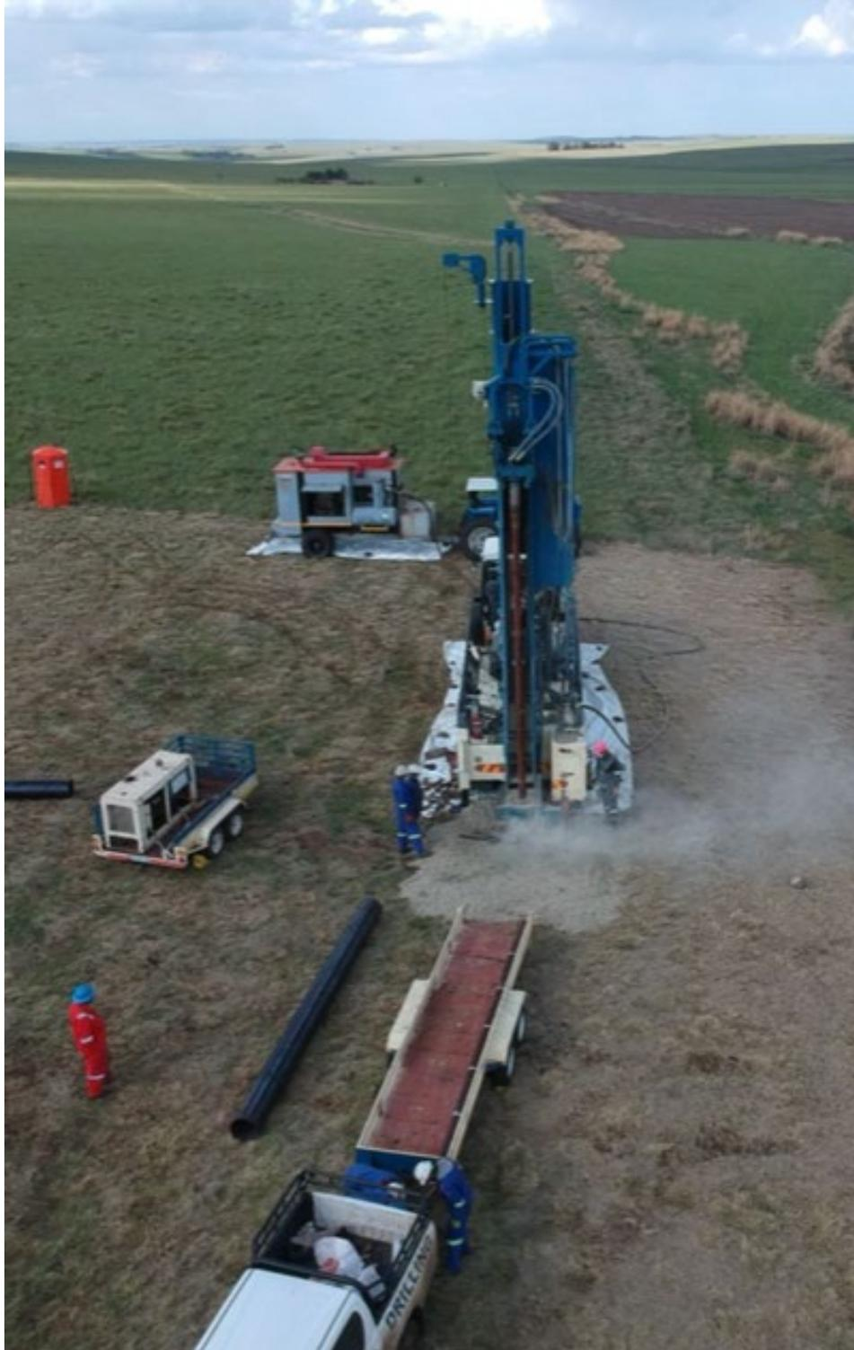
Figure 2: The B21 drilling rig spudding Korhaan 3
