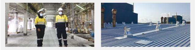
During the year work was undertaken to reduce room temperatures in the product finishing area of the Lynas Malaysia plant, by improving natural ventilation and installing new roofing and roof turbine ventilators. These changes were effective in reducing the heat impact on staff by lowering indoor temperatures and this work remains a focus of our continuous improvement program.
