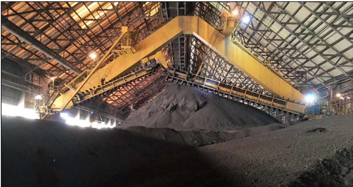
Figure 11: Reclaiming of stockpiled concentrate in the Karumba storage shed for loading onto the MV Wunma
