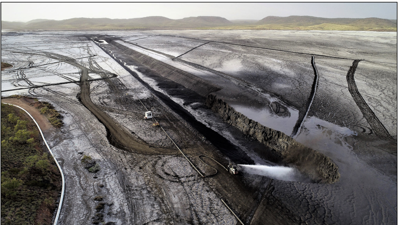
Figures 9 & 10: Overview of hydraulic mining progress at the Century Mine
