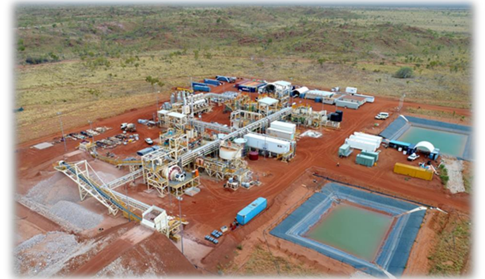
Browns Range Pilot Plant
