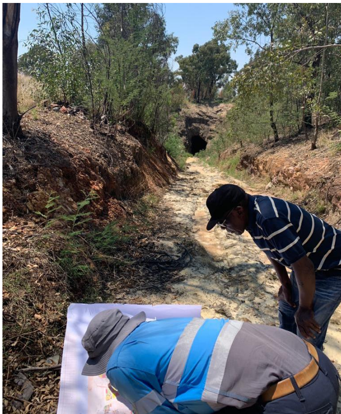
Image 2 – Newly appointed General Manager of Mining, Mr Sefika (right), inspecting the Qala Adit at the Kimberley East project area with WWI Geologist Seani Nethengwe. The Independent Scoping Study identifies the Qala Adit as the main access point for the first stage of development.
