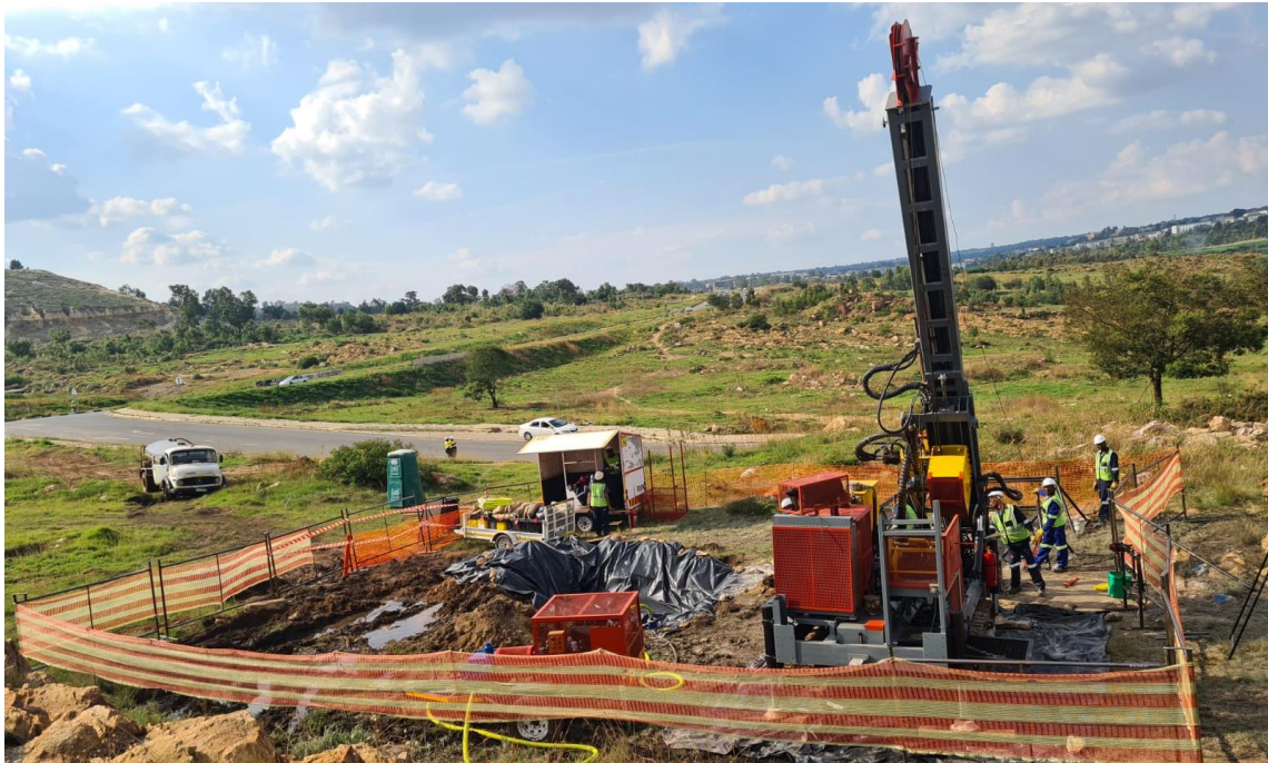
Image 1 – Drilling team commencing the 1 st of a 23-borehole diamond core drilling campaign
