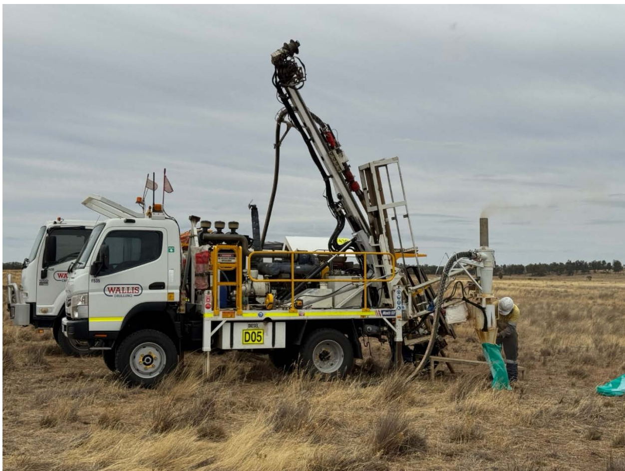
Figure 1. Wallis Drilling AC drilling rig operating at the East Peak Hill Prospect.
