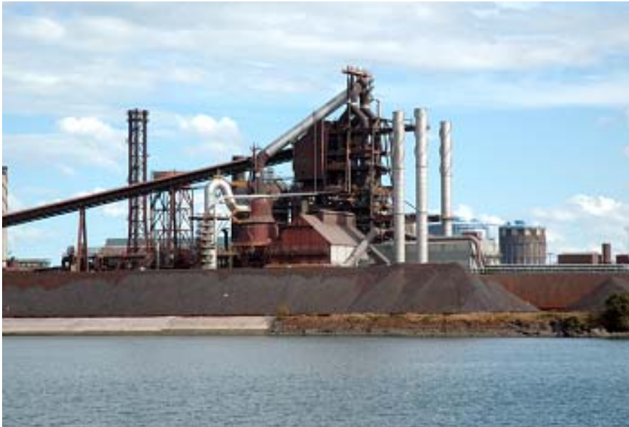
No.5 Blast Furnace
