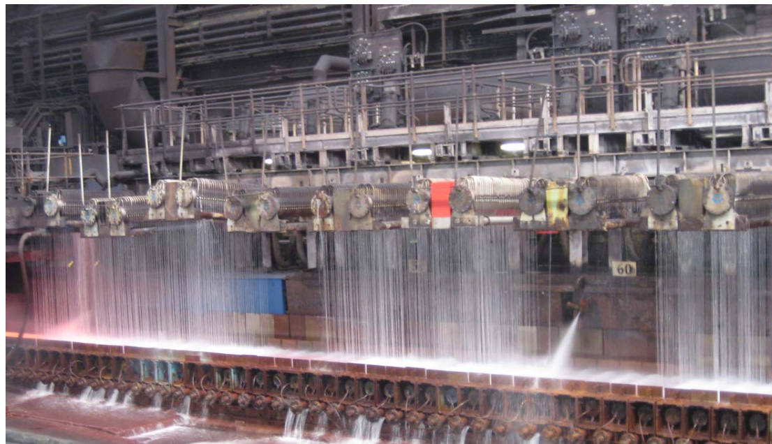
Hot Strip Mill run out table uses recycled water
