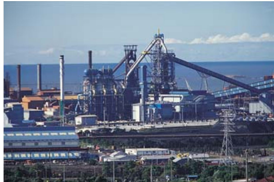
No.6 Blast Furnace
