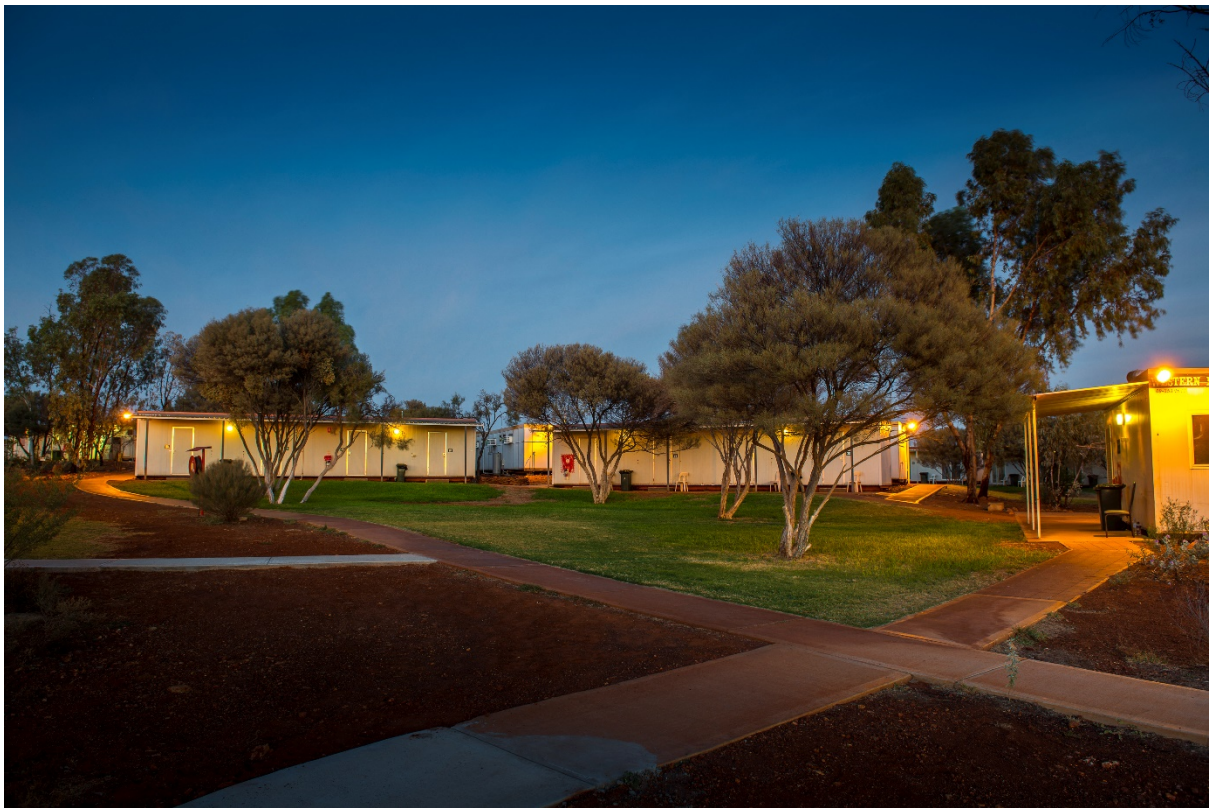
Figure 3: Rosslyn Hill Accommodation
