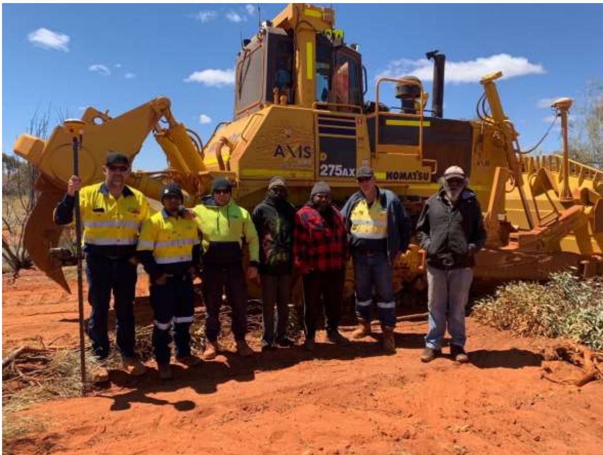
Figure 9: PRG workers, Martu monitors and earth moving machinery
