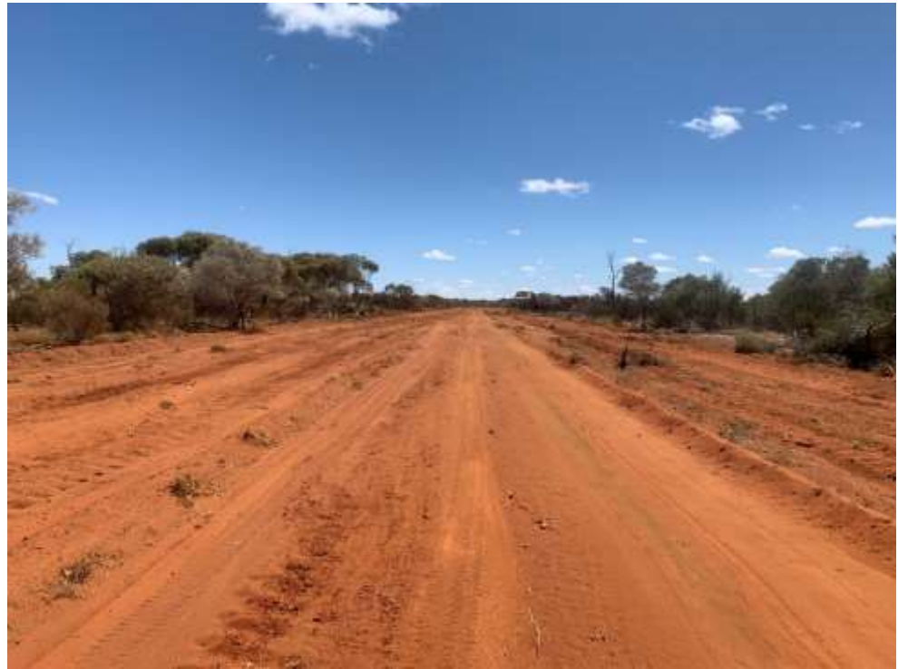
Figure 8: Northern Haul Road Clearing
