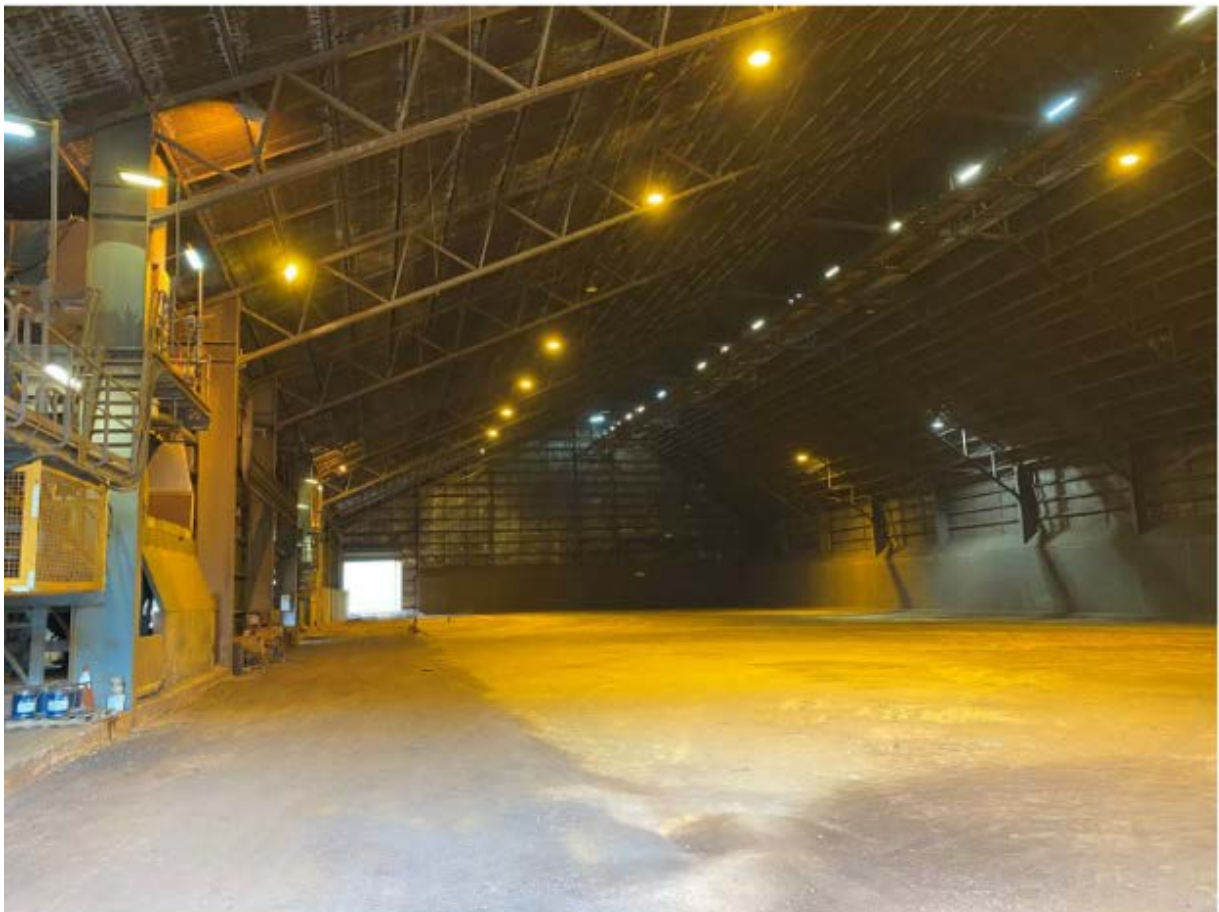
Figure 3: Site 88 - Internal Shed View
