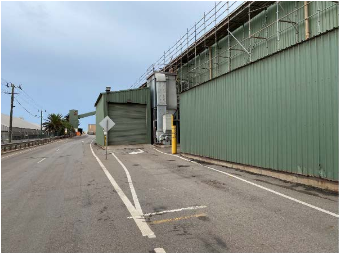
Figure 4: Site 88 – Truck Unloading Facility
