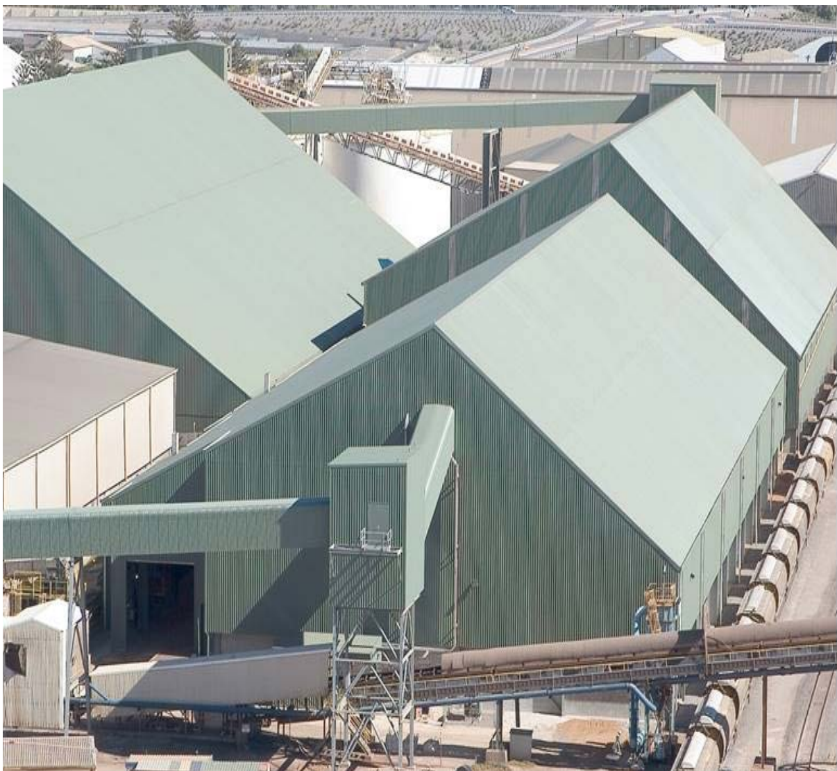
Figure 2: Site 88 Storage Shed – Aerial View
