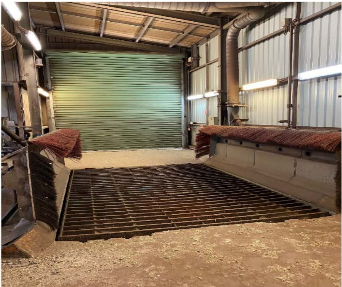
Figure 5: Site 88 – Internal View of Truck Unloading Infrastructure
