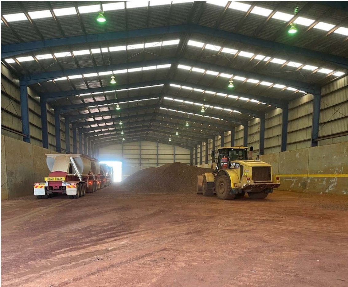
Image 2: 15,000 tonne transfer station to facilitate continued ramp-up.
