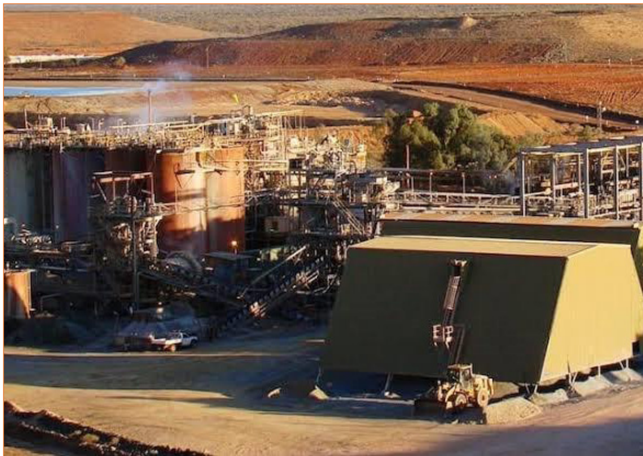
Figure 3: Blackham Resources Matilda Processing Plant Located at Wiluna.
