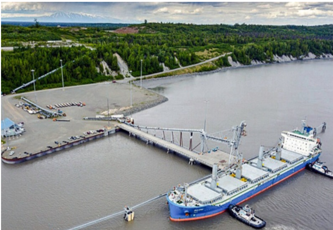
Figure 4. Photo showing the Port MacKenzie infrastructure
