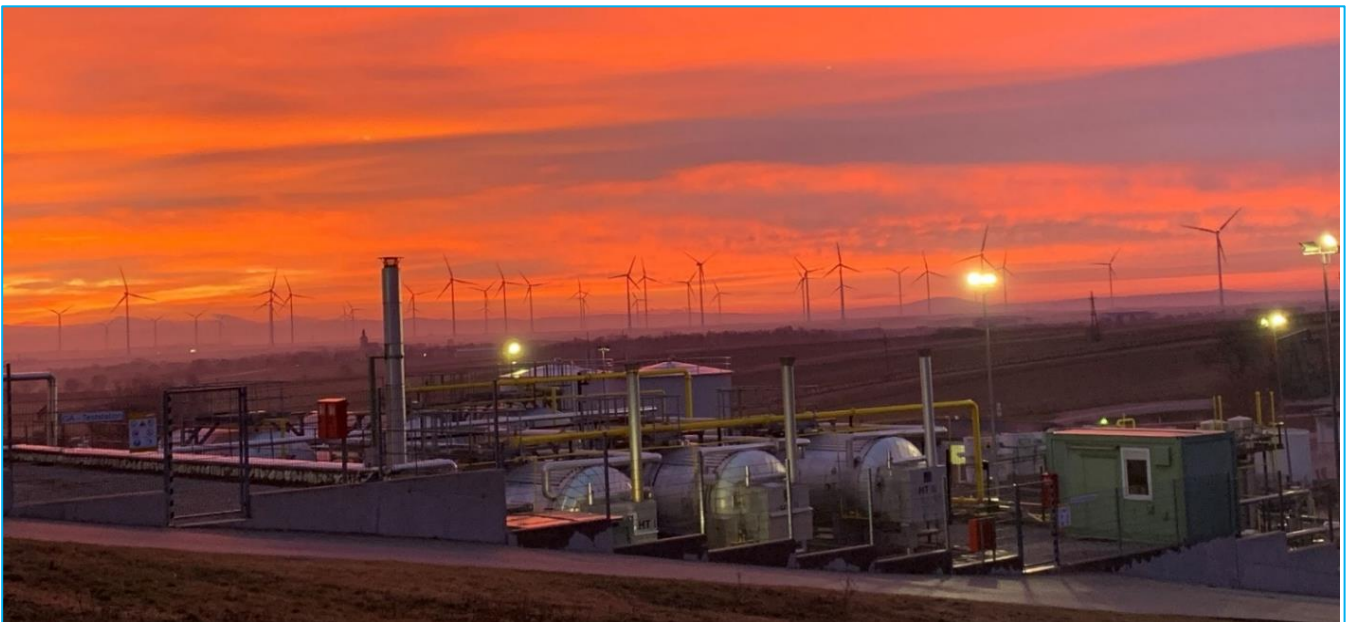
Photograph showing ADX Gaiselberg and Zistersdorf Field infrastructure proximal to the largest wind farms in Austria suitable for generating green hydrogen
