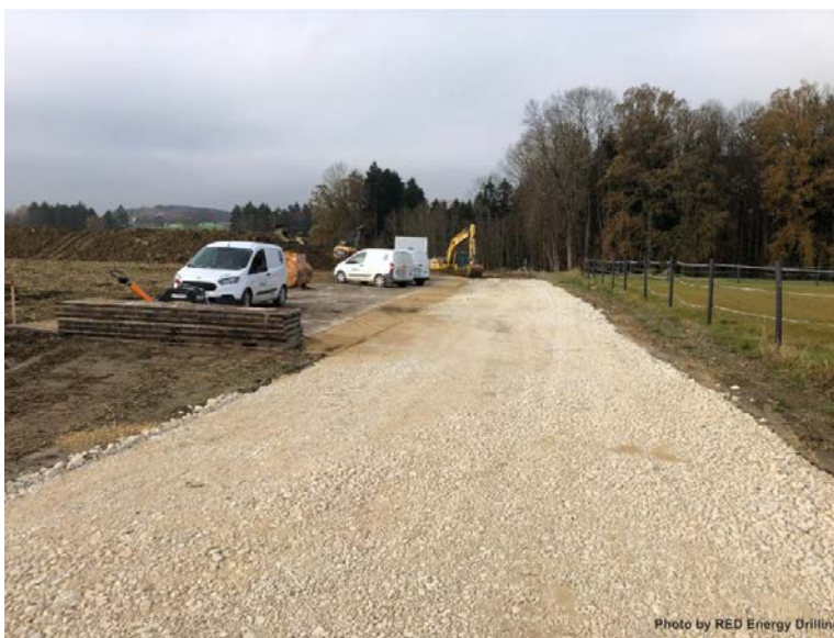
Figure 1: Anshof well site access road construction
