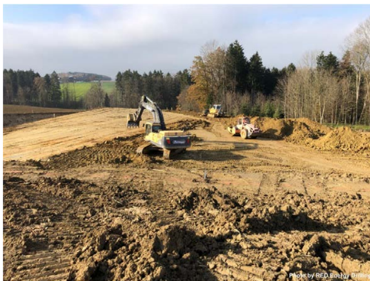
Figure 1a: Anshof main well site construction
