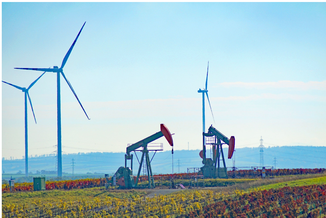
Production operations at the Gaiselberg and Zistersdorf fields in Upper Austria
