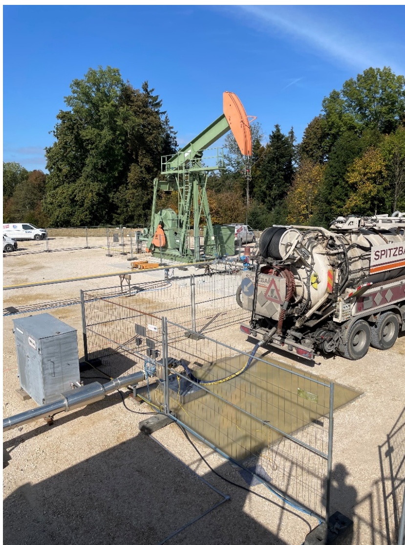
EPU installation work at the Anshof-3 location
