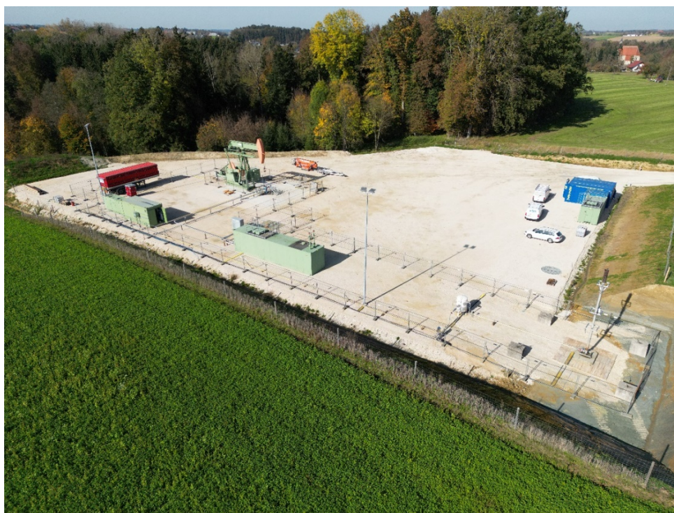
Figure 2: The Anshof-3 well and early production unit
