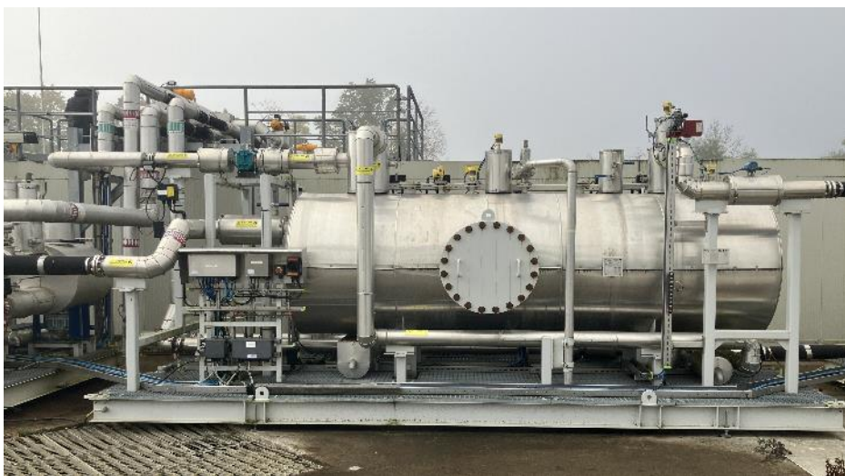
Permanent production facility (to be installed at Anshof location)
