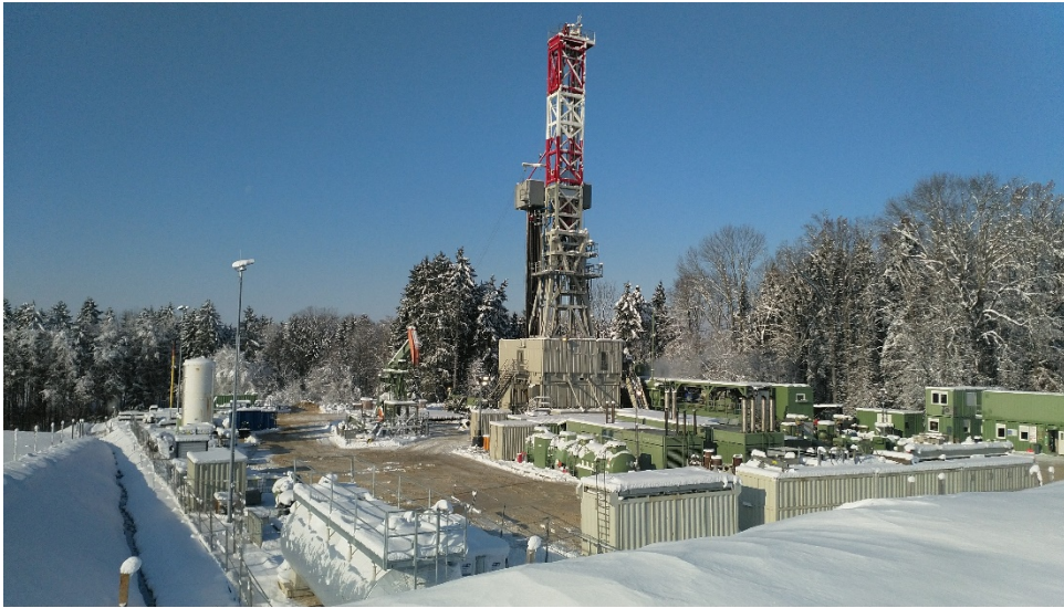
Drilling operations at Anshof-2 with the RED E-202 drilling rig. The pump jack in the back ground is at the Anshof-3 production well.
