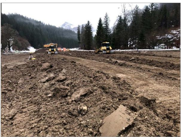
Well construction operations clearing top soil before installation of foundation material for drilling at the Welchau-1 well site
