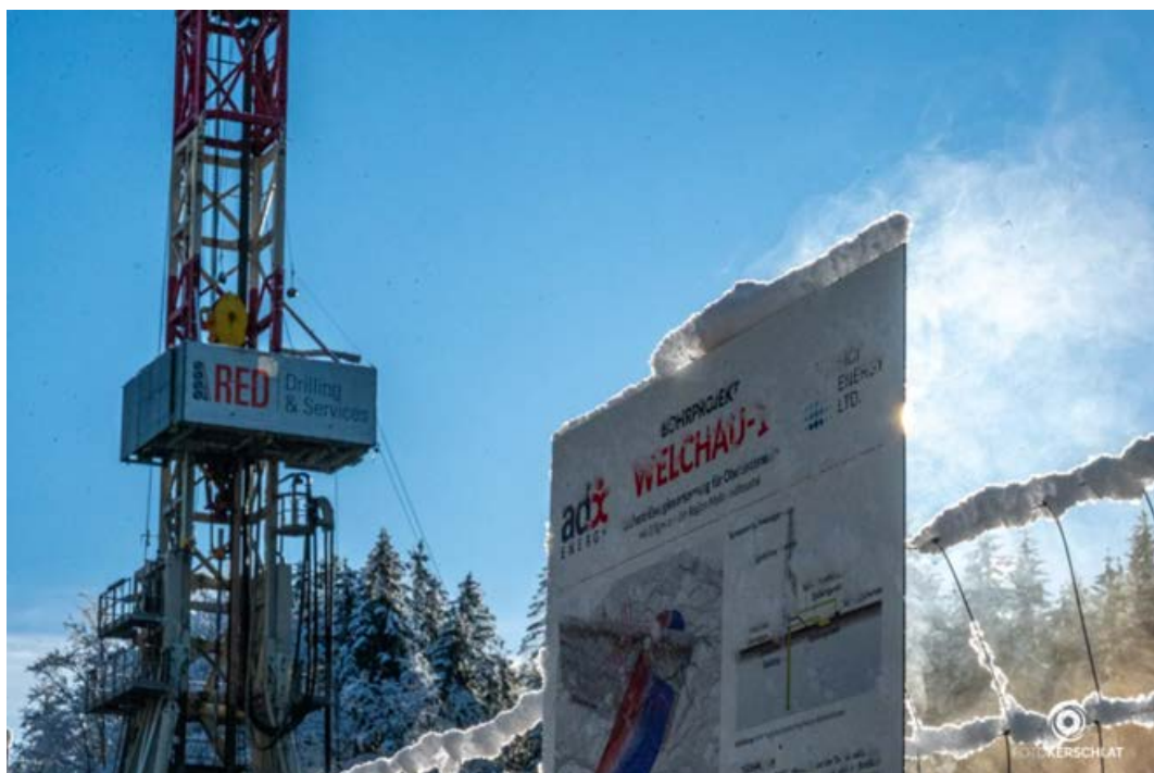
RED E200 drilling rig operations at the Welchau-1 location
