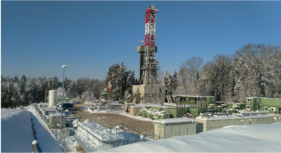
Anshof-2 Drilling with the RED E-202 drilling rig
