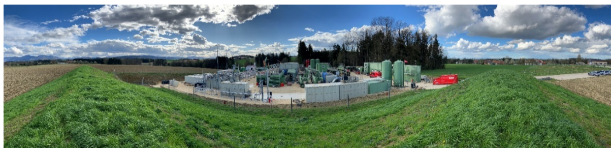
Anshof Permanent Production Facility at ADX' Anshof-3 location
