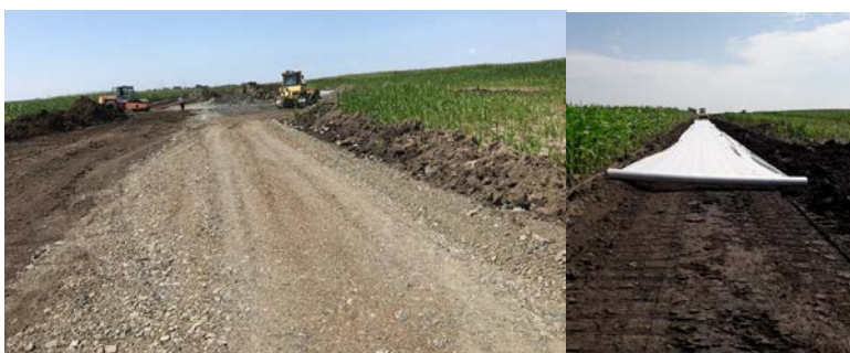
Well Access Road Construction – showing road completion and membrane (geotextile)
