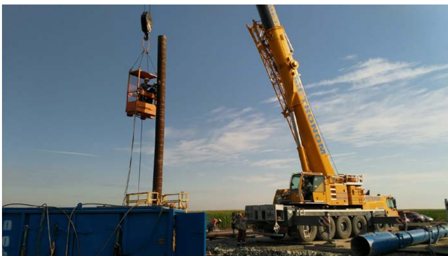
lecea Mica – 1 Well Conductor Casing Installation
