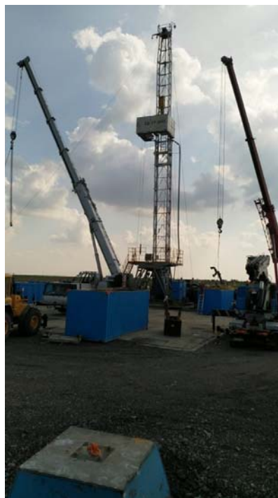
Tacrom Futura Rig 6 Assembly Operations
