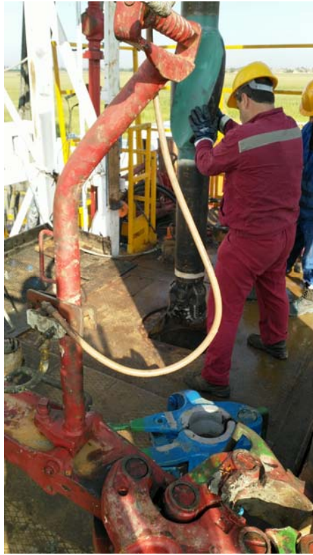
Tacrom Futura 6 Rig Floor - Iecea Mica 1 Well Preparing to Spud
