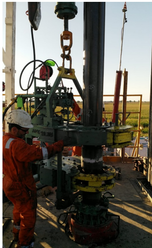
Making up and running 9 5/8" Casing
