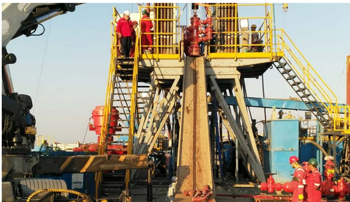
Drilling operations on the IMIC-1 appraisal well.
