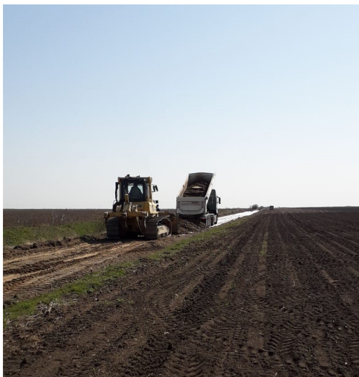
Road construction operations for the IMIC -2 appraisal well.
