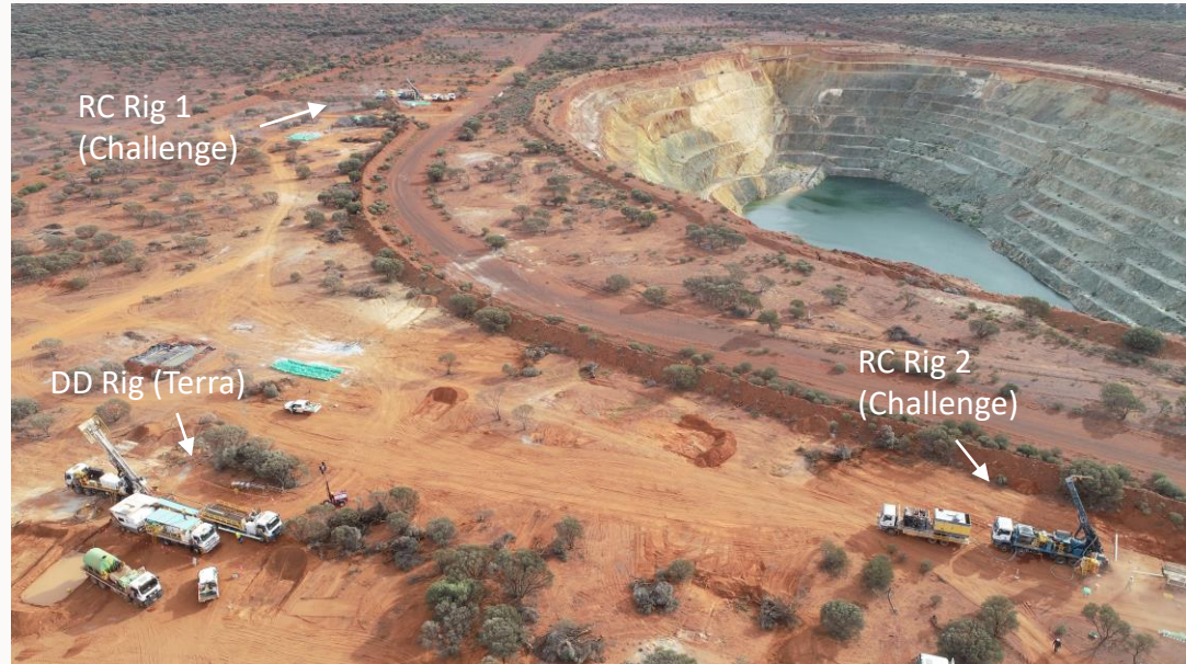
3 Rigs (2 x RC and 1 x Diamond) drilling at Lord Nelson
