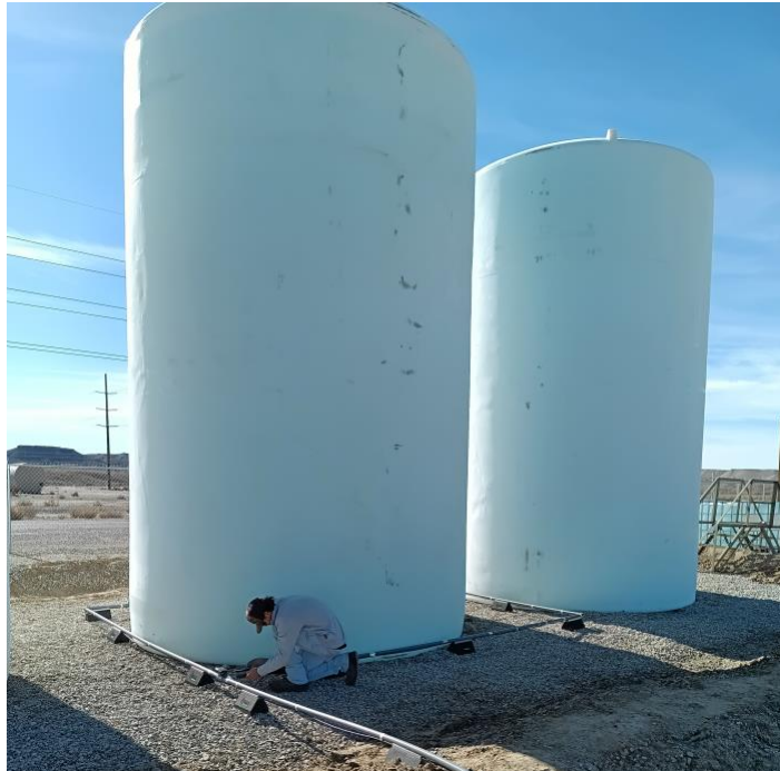
Figure 2: Two full tanks containing 32,000 gallons of lithium eluate processed by the Koch DLE at Green River, Utah, USA
