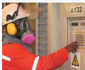
Programmable logic controllers help operators maintain optimum levels of alumina and terminate anode effects in cells at the Mozal aluminium smelter in Mozambique. This reduces emission of perfluorocarbon compounds, which are powerful greenhouse gases.
