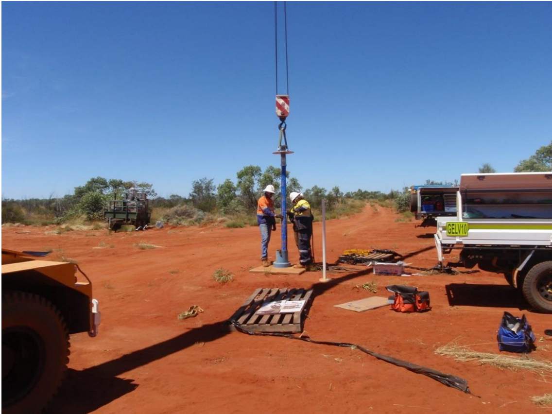
Figure 10: Bore fit out at Borefield D
