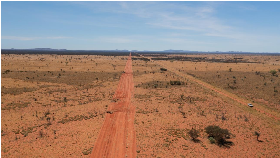
Figure 13: Pipeline corridor with Amadeus Gas Pipeline in parallel
