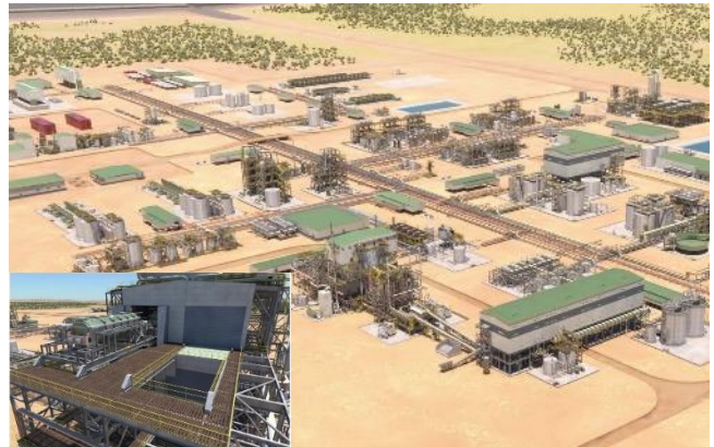
Figure 2: Pre-leach and sulphation (inset: sulphation bake unit)
