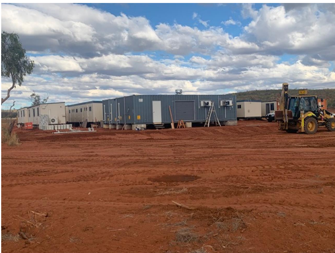
Figure 9: Fly camp under construction
