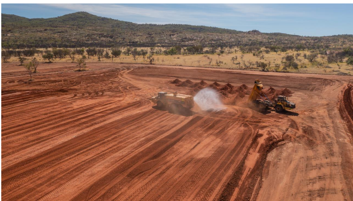
Figure 7: Village area bulk earthworks construction
