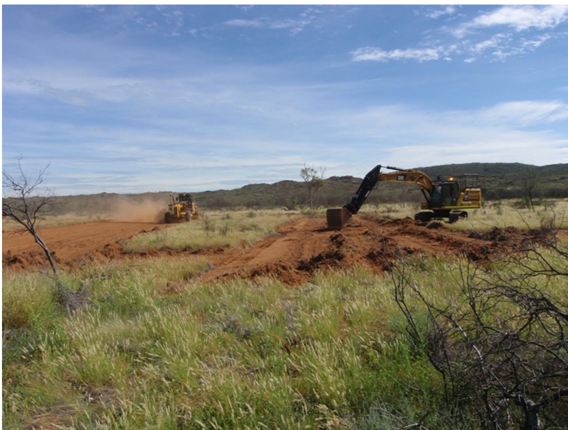
Figure 6: Commencement of clearing and civil works at the village site
