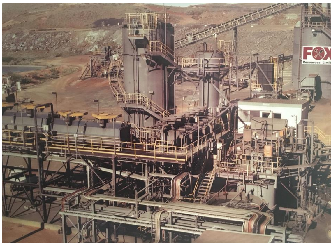
Figure 3: AGIP Radio Hill Nickel/Copper Operations (Fox 100%) - Radio Hill 425,000 tpa Treatment Plant and floatation circuits.
