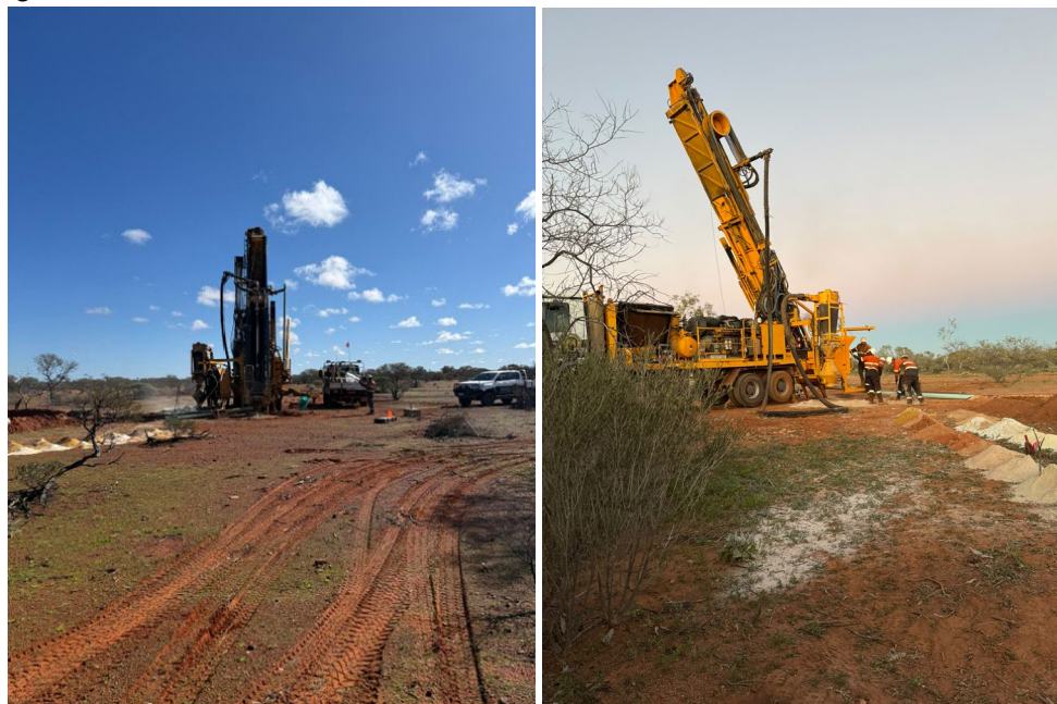
Figure 1: RC Drilling in progress
