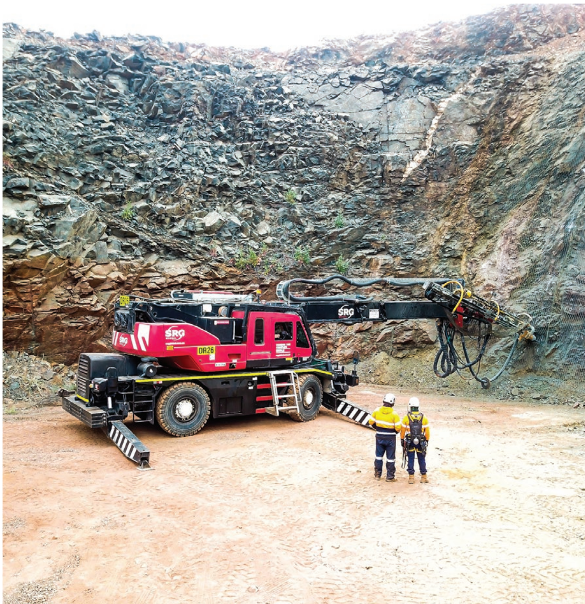
High reach drill in Paris Pit installing ground support for the new portal to be established.
