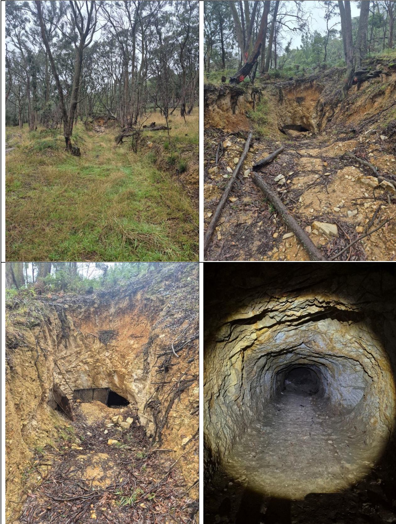
Figure 2: Photos of the existing Sister Rose boxcut, portal and adit – all looking North.
