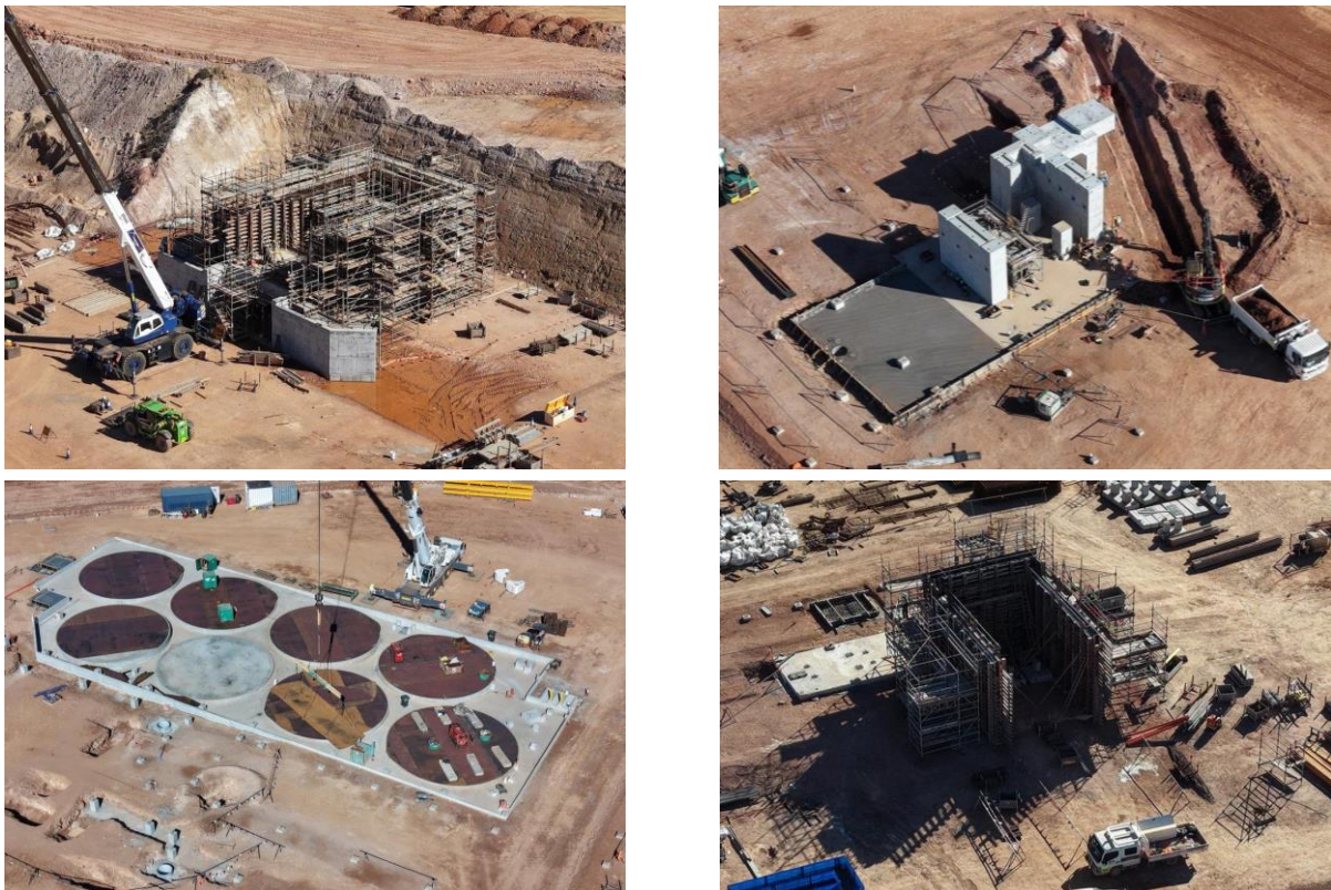
Figure 3: Construction activities underway (August 2026)
