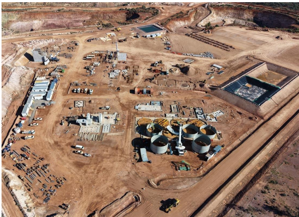
Figure 2: Laverton processing plant site (September 2026)
