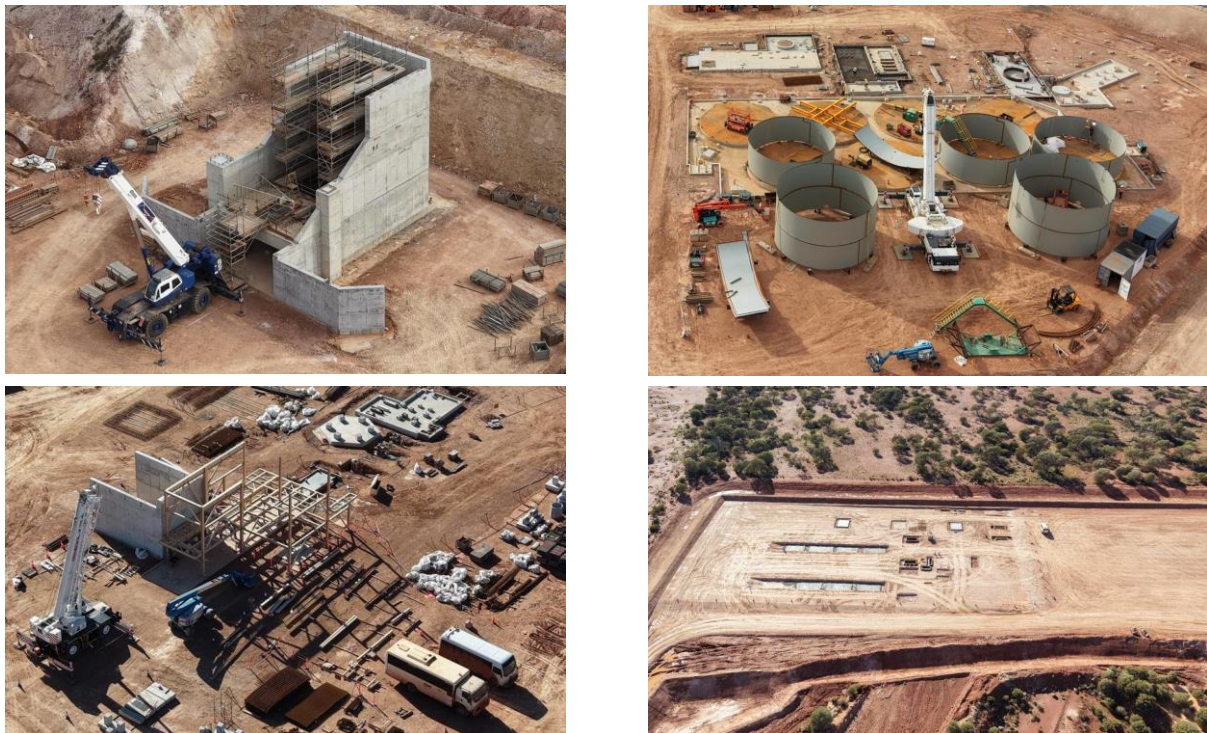
Figure 4: Construction activities underway (September 2026, reported post quarter-end) Top: Primary crusher, final pour completed (L); CIL circuit, tank construction underway (R) Bottom: Surge bin area, structural steel erection commenced (L); power station area, concrete commenced (R)
