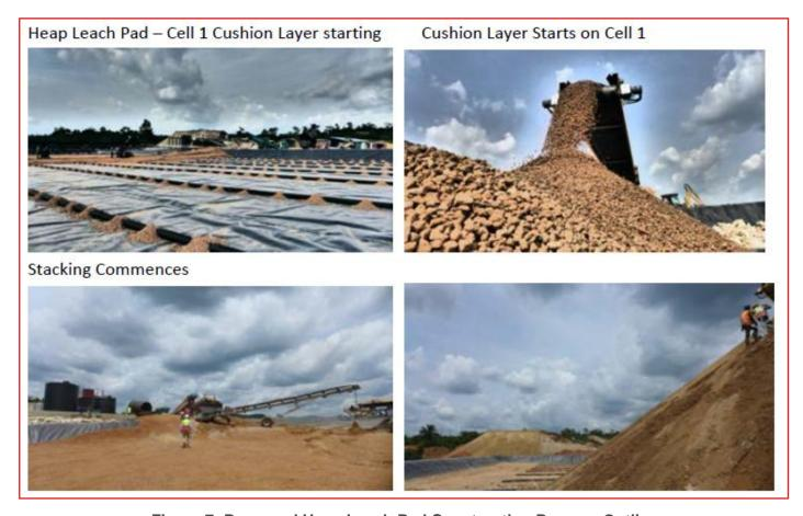
Figure 7: Proposed Heap Leach Pad Construction Process Outline
