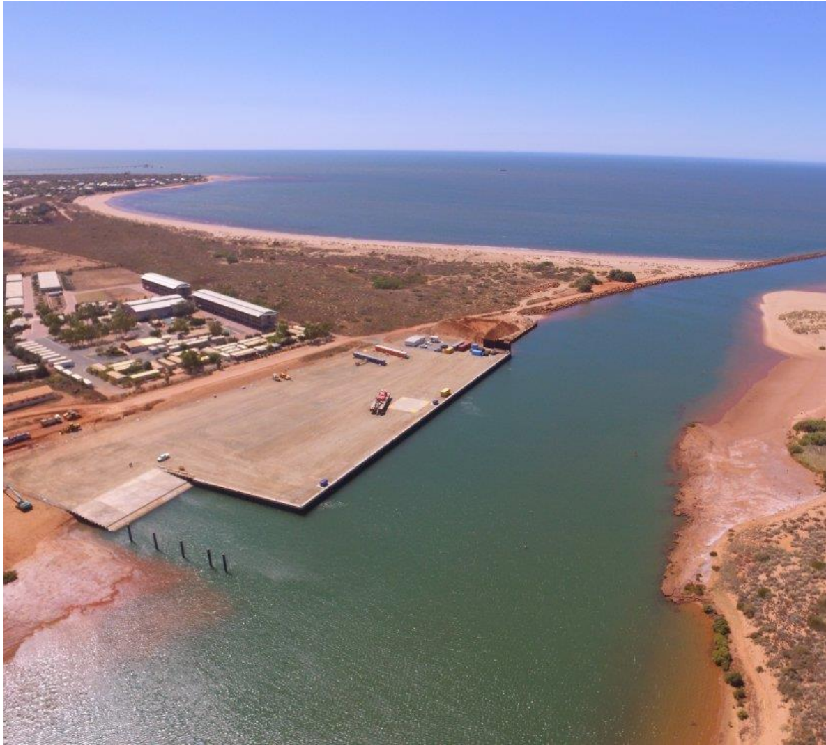
Figure 2 Oblique aerial view of the OMSB Facility at Beadon Creek near Onslow showing the dock-side hardstand and shipping channel.
