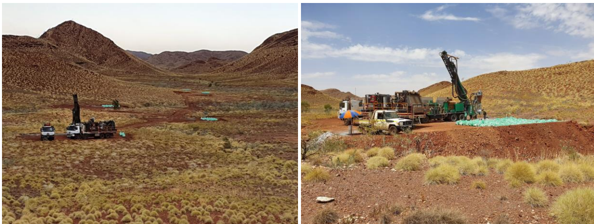
Fig 2 RC drill-rig on-site at Top Camp in late 2019.
