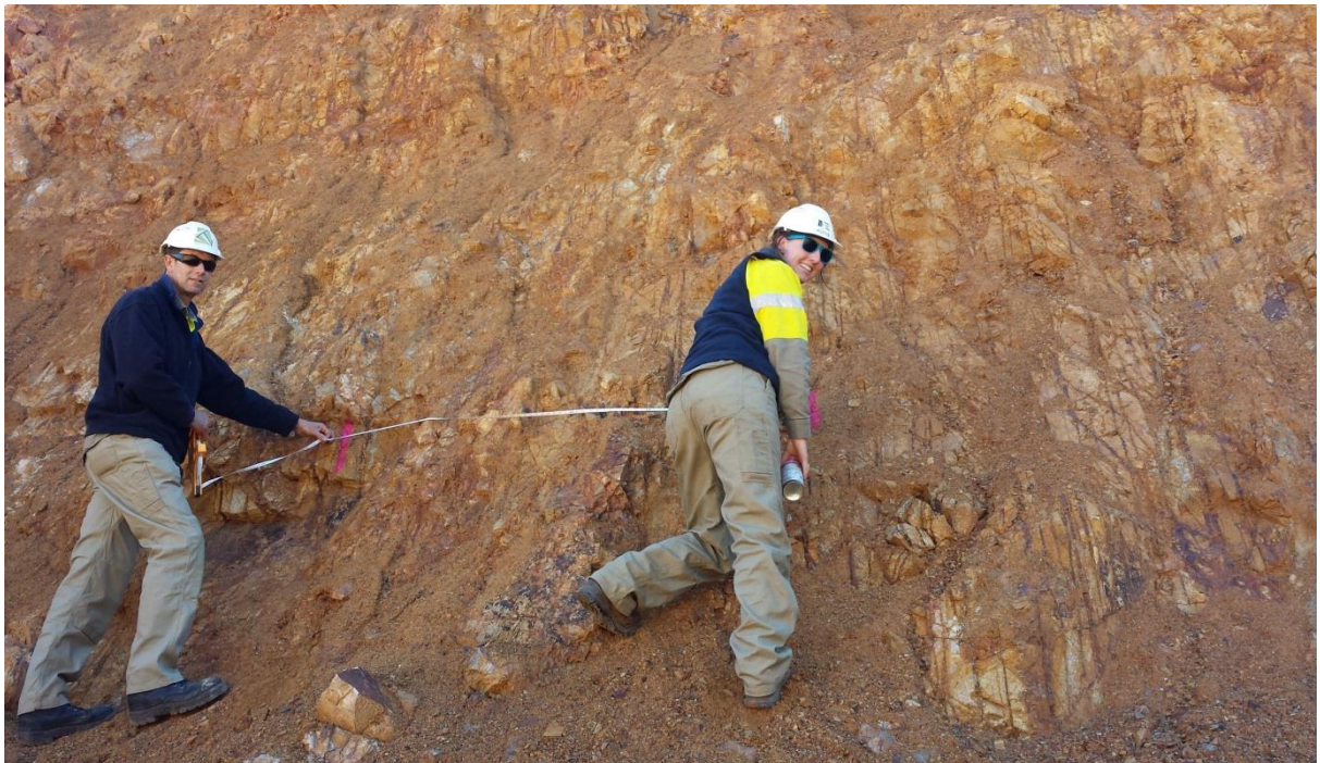
Figure 4. The face at Copper Quarry showing sets of sheeted veins (upright and dipping downwards towards the right of the photo) and iron staining, in part from weathering of disseminated sulphides.
